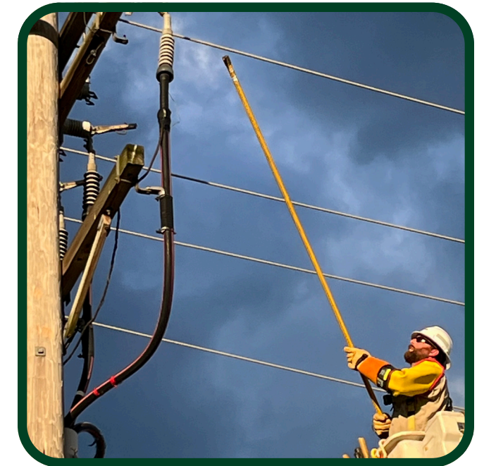
EnergyUnited lineman working to restore power during Tropical Storm Helene.
